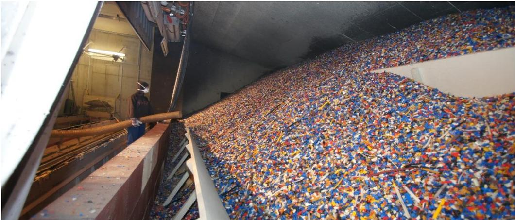
**RUTEC** R5000 can be installed across the entire area as well as in the form of a covering coat on the present sand projectile catching device. We recommend additionally installing a subconstruction to prevent the granulate from slipping and a covering tarpaulin of our natural rubber (**RUTEC** R1078) to avoid contamination by foreign substances.
